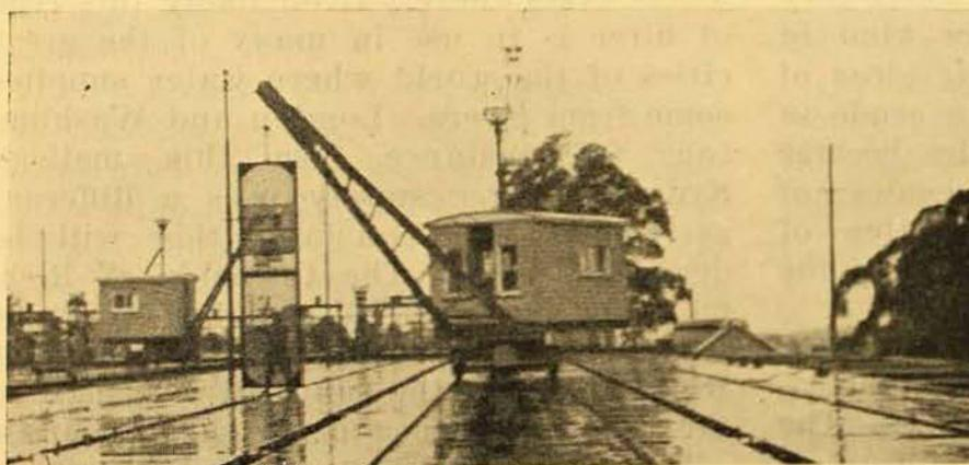
Sydney's water is purified by passing it through screens of fine wire mesh. One of these screens is seen here, hoisted from the side of the filter chamber for cleaning. An electric crane moves up and down along the side lifting the screens as required. The size of the screen may be judged by comparing it with the man's figure seen through the mesh.
