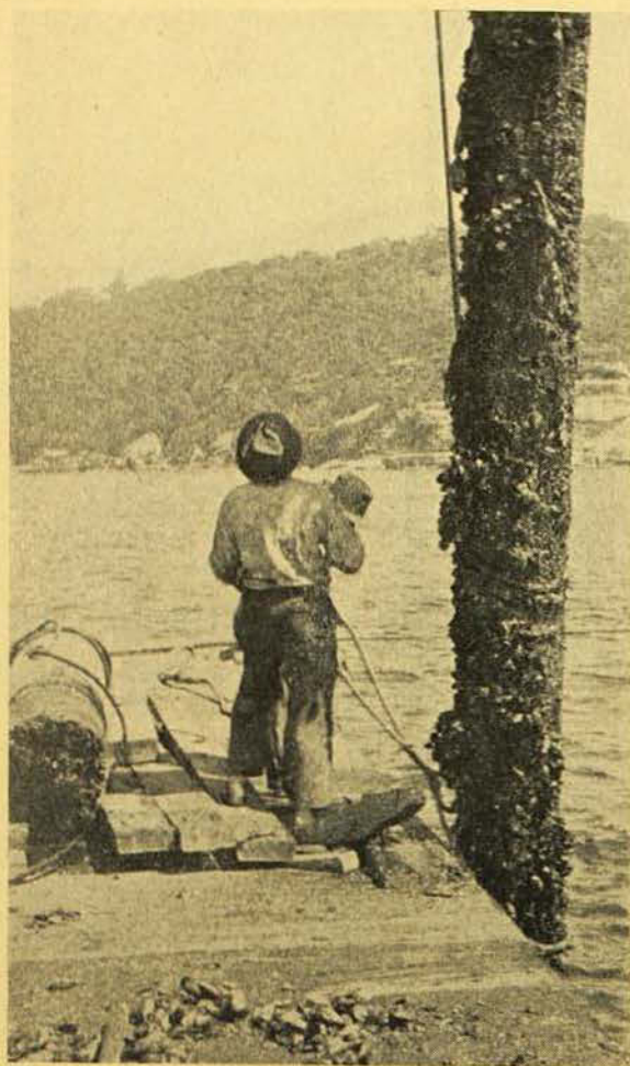
In the drawing process, one side of the pile has been scraped almost clear of growths as it ground against the side of the pontoon. Elsewhere, the thickness of the growth may be appreciated.
