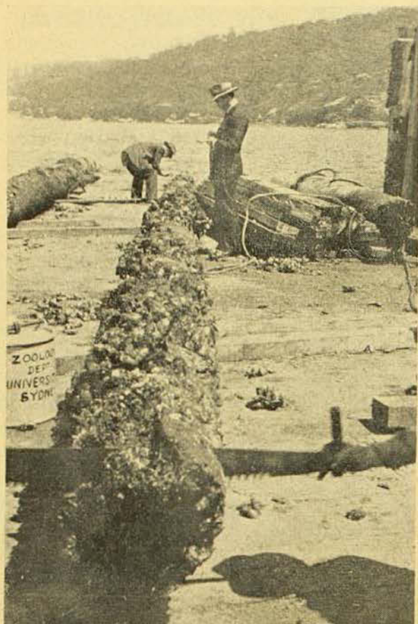
The lower sixty-five feet of the snapped pile shows the thick growth of mussels in the middle region. The remainder of the pile lies to the right of the stack of sleepers.
