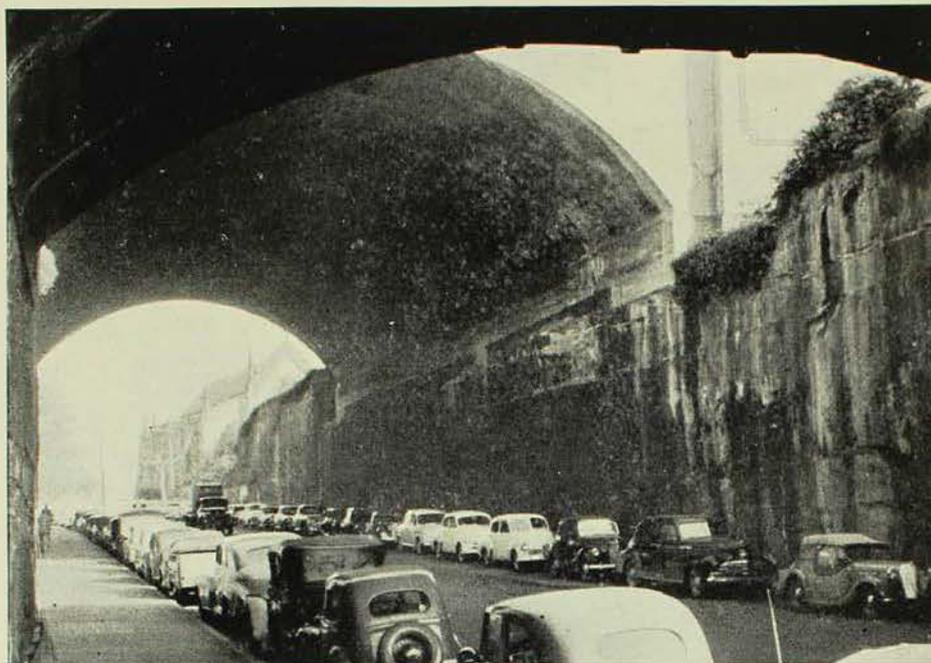
The Argyle Cut, where Argyle Street passes under the concrete arch over which traffic travels towards Sydney Harbour Bridge. The light coloured stains on the right-hand side of the cutting are the travertine formations.
