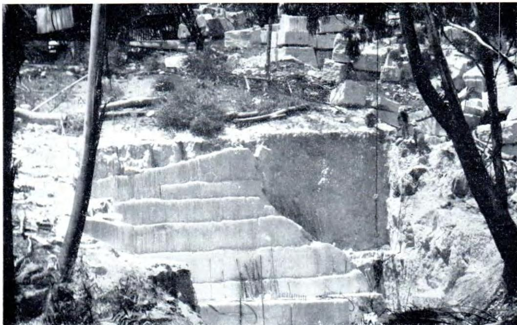
The Wombeyan marble quarry, N.S.W. Note the closely-spaced drill holes both on the quarry face and on the loose blocks on top. [Photo by courtesy of Melocco Bros.]
