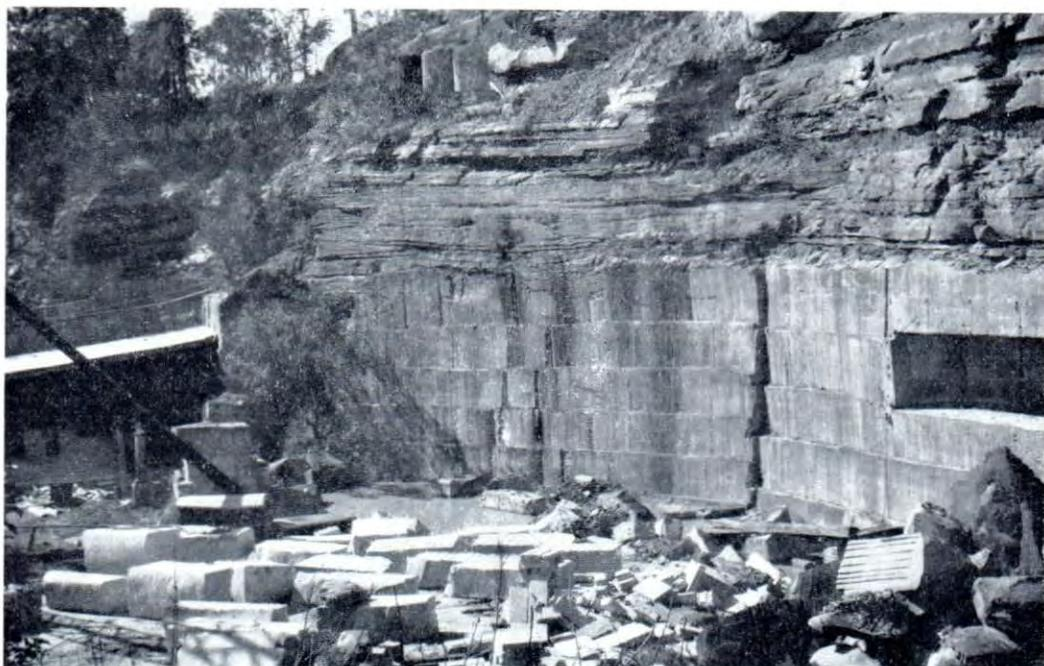
One of the sandstone quarries at Gosford, New South Wales. Note the vertical working face on the lower bed of freestone from which blocks of dimension stone are quarried. The outlines of the blocks can be seen. The overlying thin-bedded flaggy sandstone is of no use as a building stone. [Photo: Author.]
