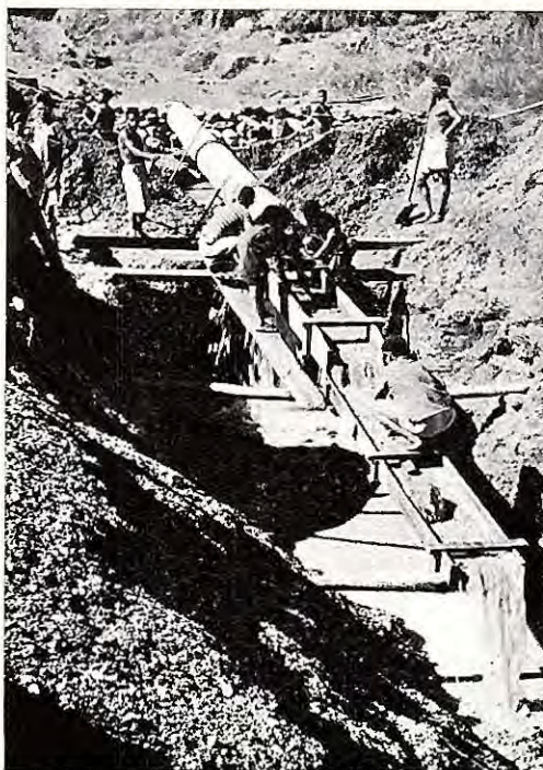
Boxing alluvials in upper Edie Creek. [Photo: Bureau of Mineral Resources.]
