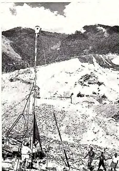
Deep alluvials being tested with a percussion drill at Koranga, Wau. The Koranga open-cut alluvial workings are in the background. [Photo: Bureau of Mineral Resources.]
