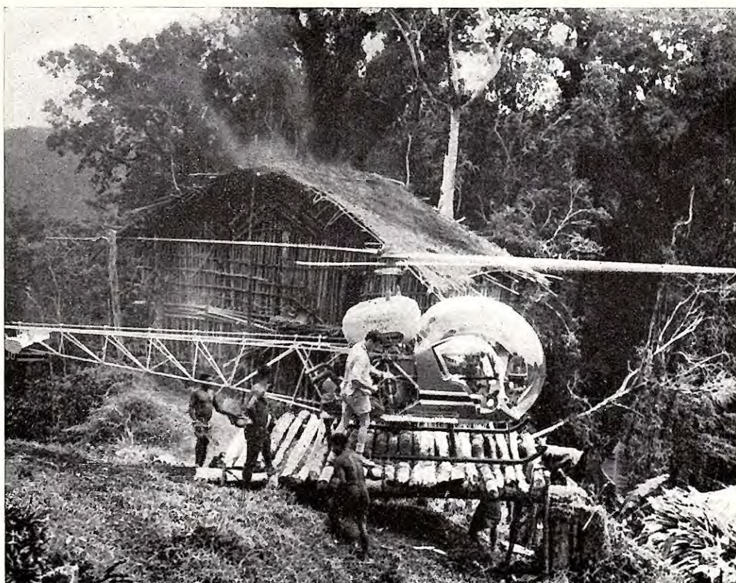
Figure 2.—A helicopter pad constructed by a Bureau of Mineral Resources traverse party (one geologist and five carriers) at the end of a week-long traverse in the headwaters of the Salumei River, South Sepik region. It was not always possible to find clearings at the end of a traverse, and often a full day's work was required to clear a pad in virgin forest. The hut belongs to the Bikalu people, who had never before been visited by white men. [Photo: Bureau of Mineral Resources.]
